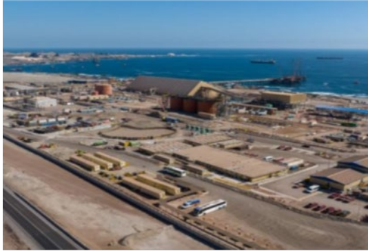
QB desalination plant
