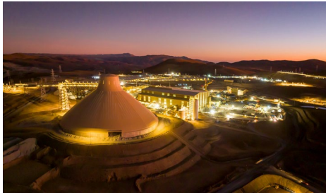
Copper Operations Top 10 copper producer operating in the Americas
