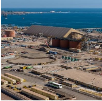
QB desalination plant.
